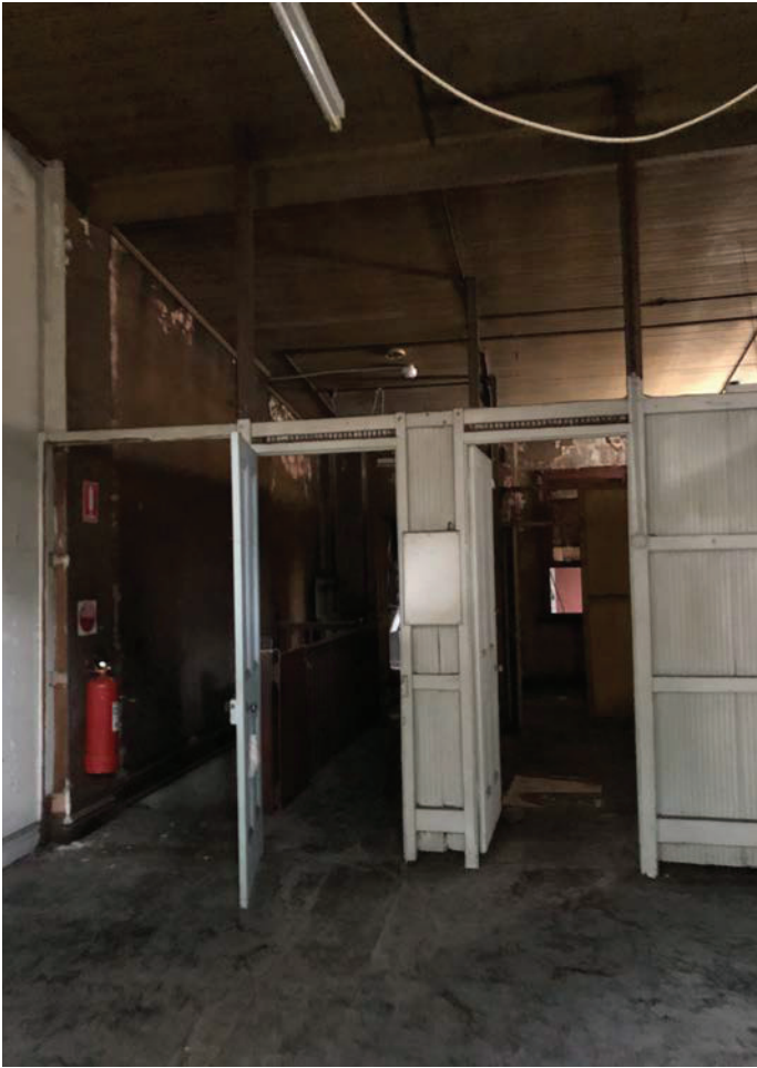
Figure 9: Second floor partitions, 84 Dixon Street.
