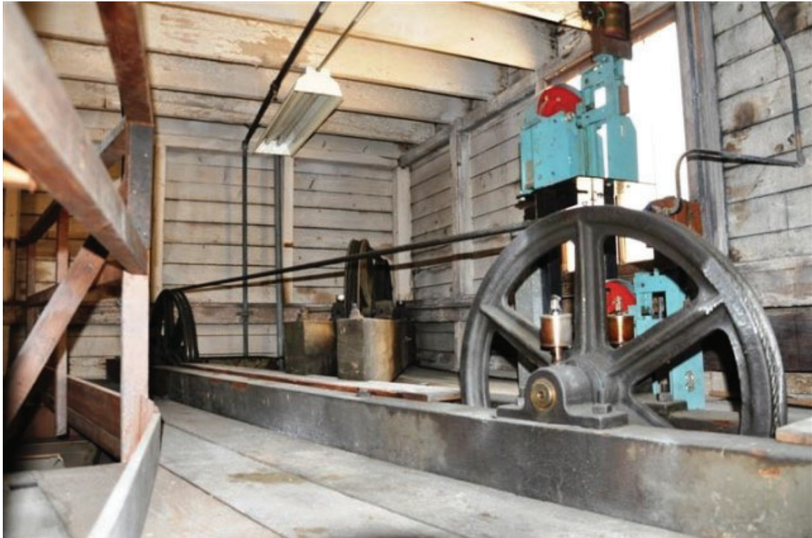
Figure 5: Hydraulic lift cable room (Source: 'Former Shelley warehouse including interiors, NSW Heritage Inventory)
